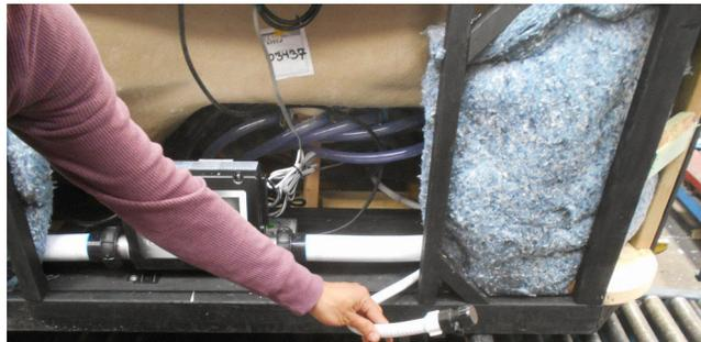
Pictured to the right is the inside of the spa behind the front door. The electrician now has access to connect the spa for power. While the front door is off, refer to page 10 for instructions on ensuring the plumbing fittings are secure (but do not be tempted to over-torque or over-tighten these fittings).
