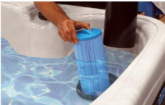
Unscrew the cartridge and remove it.
