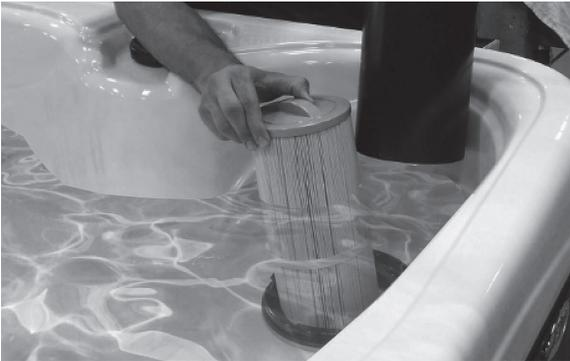
Unscrew the cartridge and remove it.
