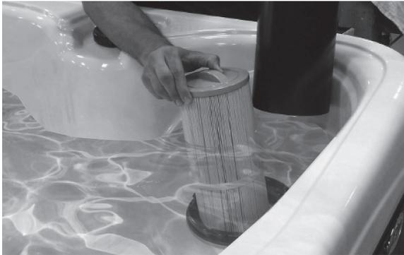
Unscrew the cartridge and remove it.
